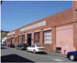
fitzroy rose street fitzroy rose street 144 unit 1
