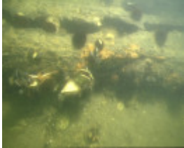
S125 CityOfMelbourne PortPhillipBayPointHenry StructureDetail
