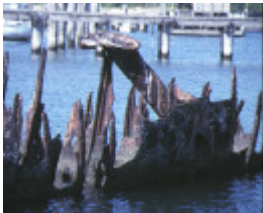
S384 J7Submarine PortPhillipBayHampton Structure
