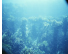
S612 Schomberg PeterboroughCurdiesInlet InletPosts
